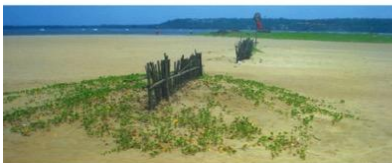
Sand dune restoration initiative using sand fence at Miramar beach.
