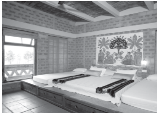
Bricks for the rooms were made from excavated mud from the site
